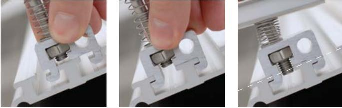
2. Turn the screw 2-3 times (up to the marking line). By doing so, the DICONAL® - system clamp is secured from falling out - its position may still be varied to the left or right towards the solar module. A spring integrated in the DICONAL® - system clamp helps positioning the modules by retaining the middle clamp sufficiently upright.
